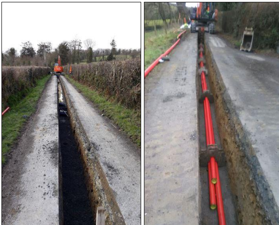
Figure 3.5: Typical Trench Construction for Electricity Lines within the Public Road
