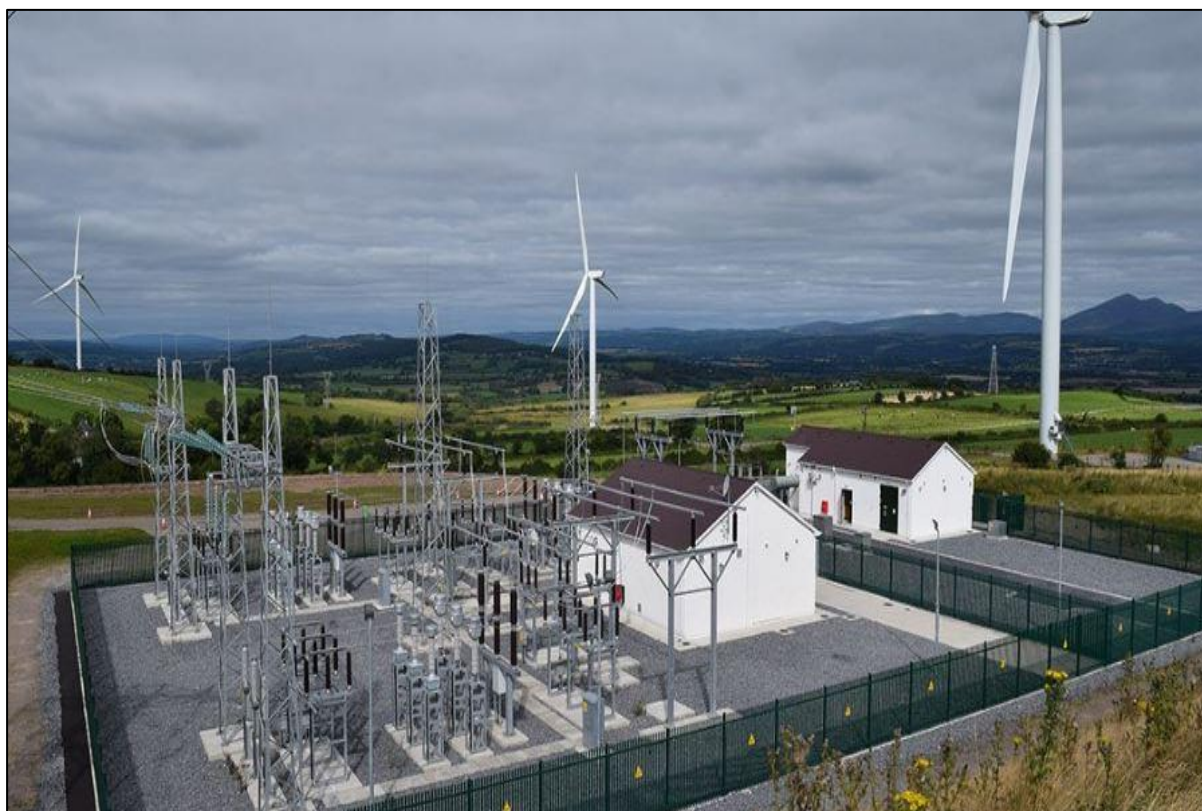
Figure 3.2: Example of a typical 110kV AIS Substation
